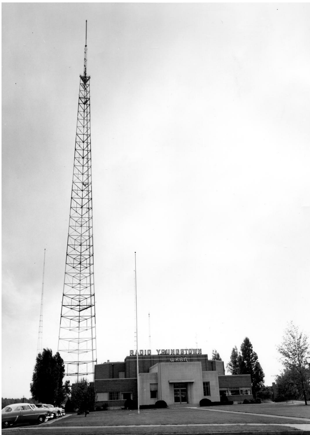
Figure 14: WKBN's Radio Youngstown and television tower at Sunset Boulevard, Youngstown, circa 1953. BMAMV Collection.
