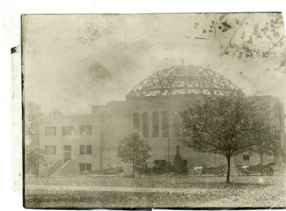
Construction of Congregation Rodef Sholom (1914) Congregation Rodef Sholom Archives
