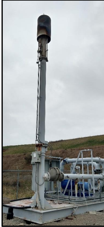
Figure 1.10: When the Gas to Energy Facility is not operating, landfill gas is flared.
