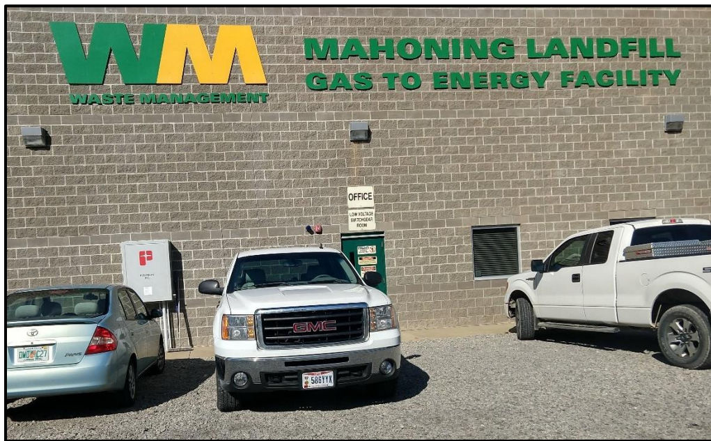
Figure 1.8: The Mahoning Landfill Gas to Energy Facility for on-site electricity generation
