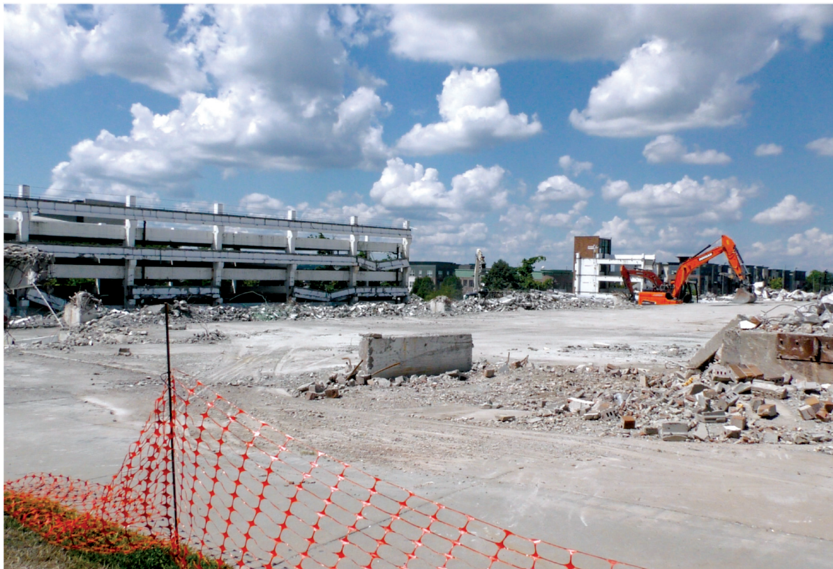
M-60 parking deck in August.
