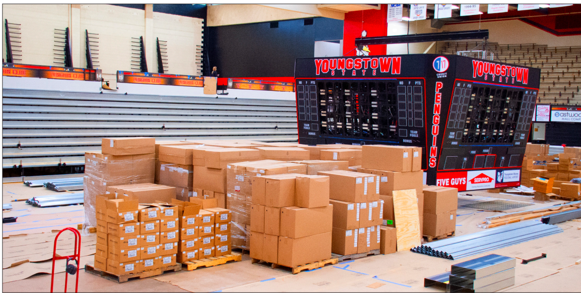
Beeghly renovations started in May and is expected to end Sept. 16.
