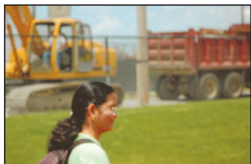
Top: Construction on University Plaza was halted during the gas leak.
