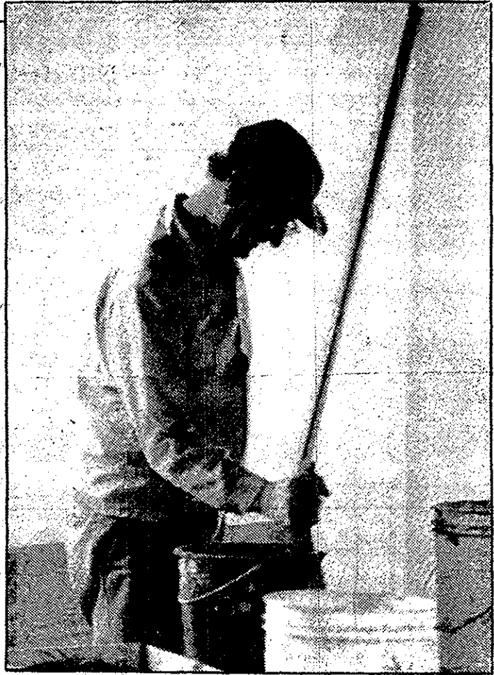
The Jambar/George Nelson A construction worker mixes plaster to be used on the walls of a former office on the first floor of the Kilcawley residence dorm. The Kilcawley offices are being remodeled to provide more space for residence hall students.
