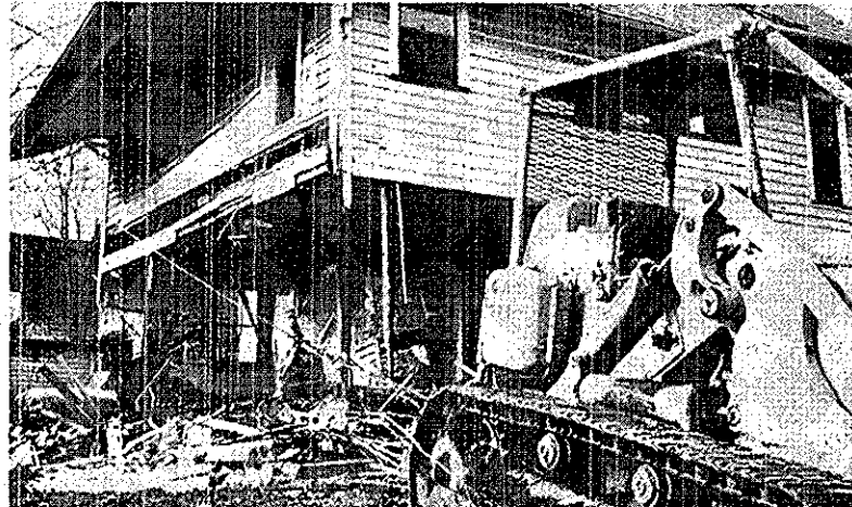
Destruction makes way for progress as the University Redevelopment program swings into high gear.
