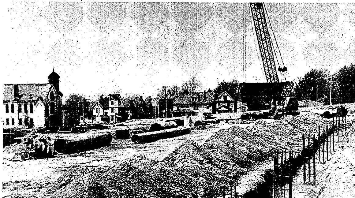
NO CONSTRUCTION - The current strike by the Operating Engineers is responsible for the halt to construction of the parking decks. Further construction of the decks will not resume until the engineers have settled.
