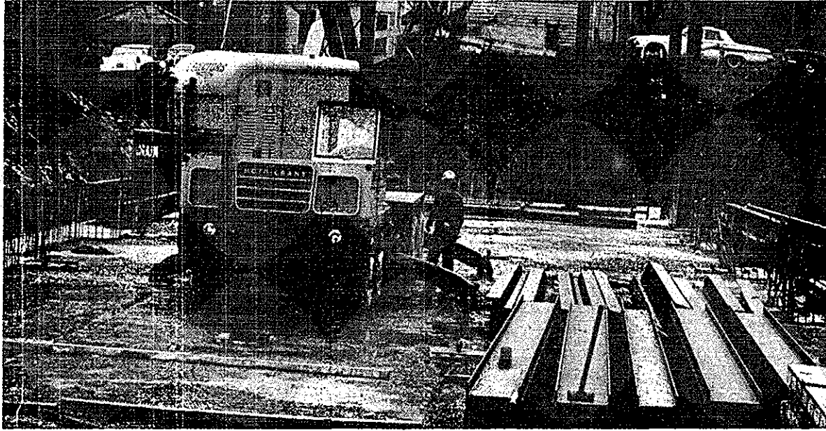
T. H. Martindale, housing director, announced last week that the Kilcawley dorm will be torn down and rebuilt from the foundation up. Martindale said the move was necessary because of the "cheap" materials used in the original building. Workmen are pictured removing the concrete foundation of the old dorm.
