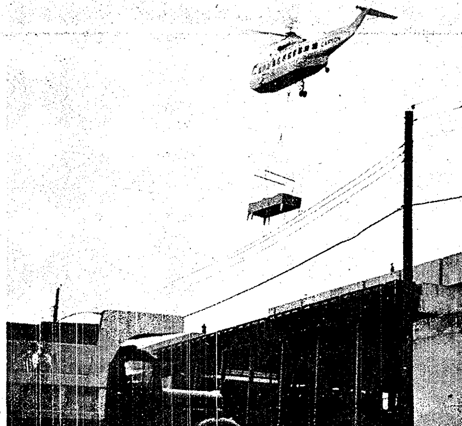
FLYING HIGH - A helicopter lowers air conditioning units on the new Beeghly Physical Education building. Scheduled completion date for the building is fall, 1971.
