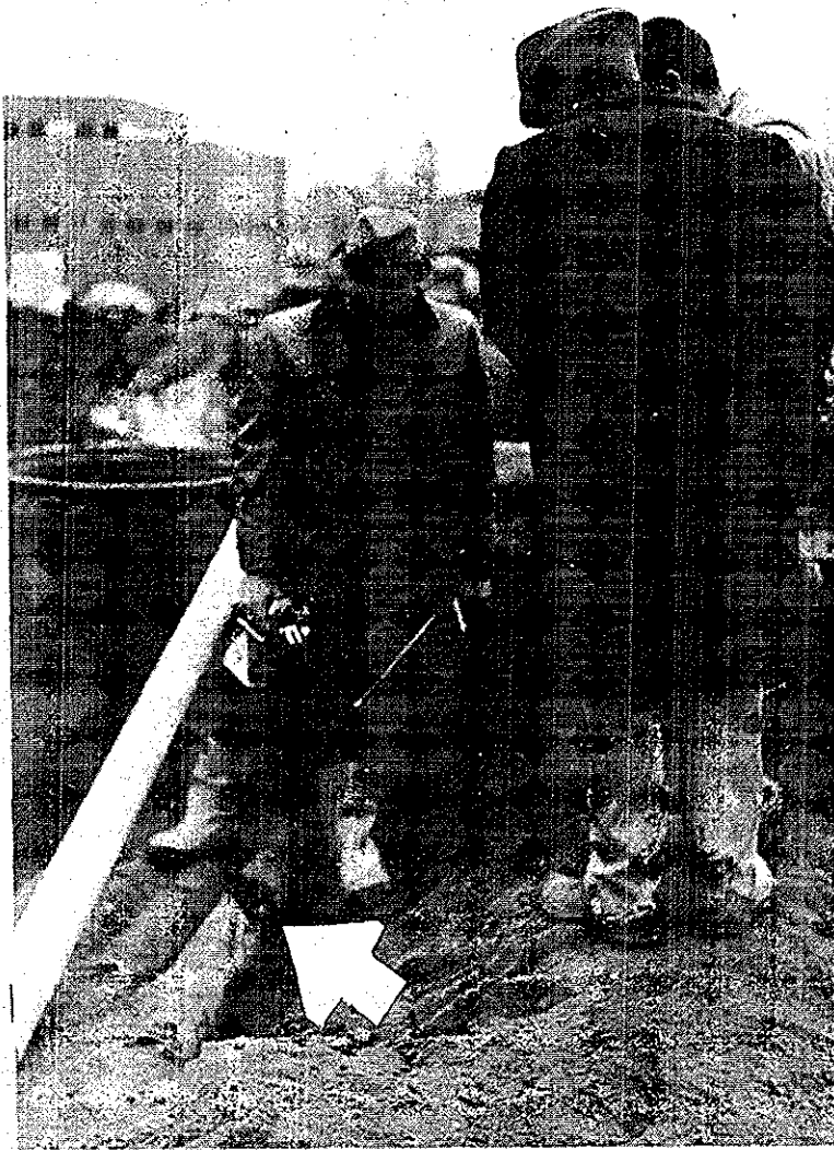
CABLE CUT —Raymond Orlando, Director of Physical Plants, and two electric company officials examine the break in the cable that caused yesterday's blackout on campus. Photo by Joe Hake.
