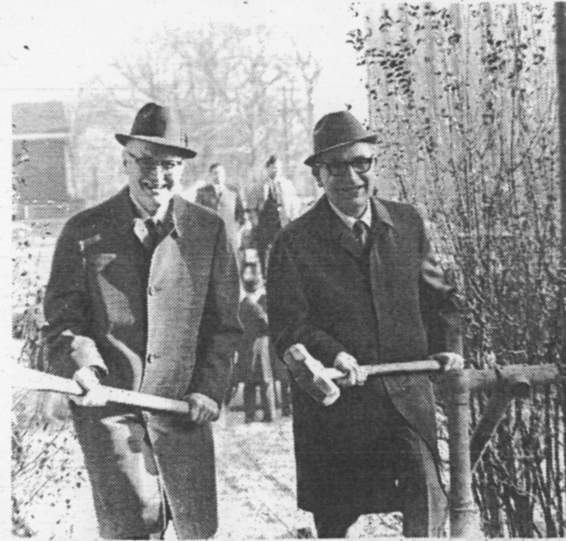
President Pugsley and Mayor Flask begin the demolition work.
