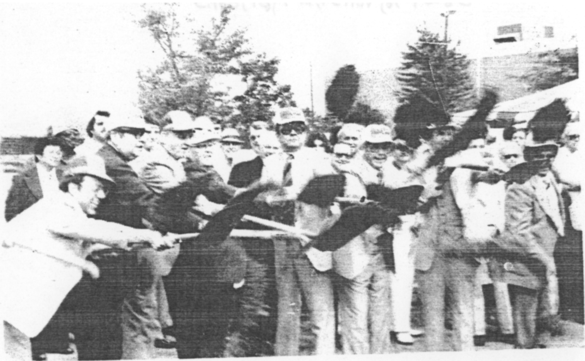
WORK BEGINS – John Carano, president of Student Government (left to right), Senator Oliver O’Kasic, Arnold Stambaugh and President Coffelt join other dignitaries in Wednesday’s Groundbreaking ceremony marking the beginning of construction for the YSU All-Sports Complex.
