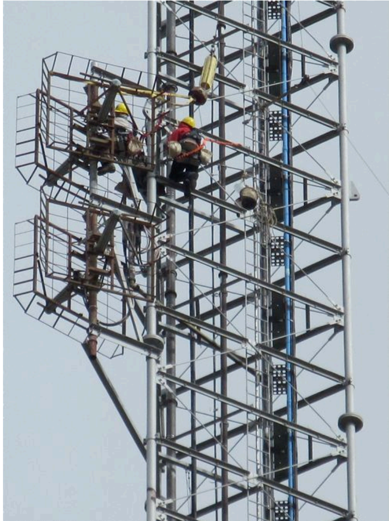
Workers install WYSU's new antenna more than 300 feet up on the south tower at the WKBN complex along South Avenue in Boardman.
